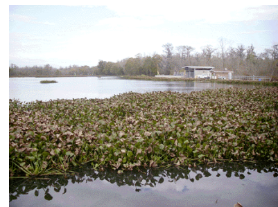
Luling Pond pump station
